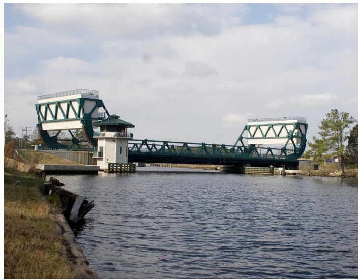
Figure 13 – Great Bridge Bridge, Chesapeake, VA
