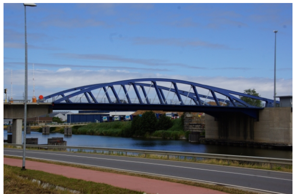
Figure 31 – Boulevard Bridge, Williebroek, Belgium
