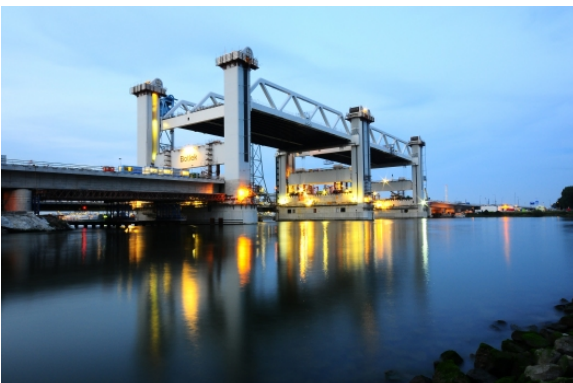
Figure 26 – Botlekbrug, Rotterdam, Netherlands
