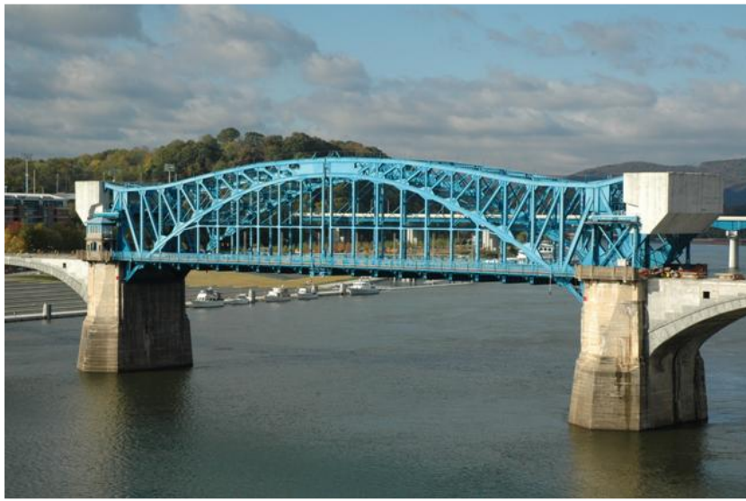
Figure 12 – Market Street Bridge, Chattanooga, TN
