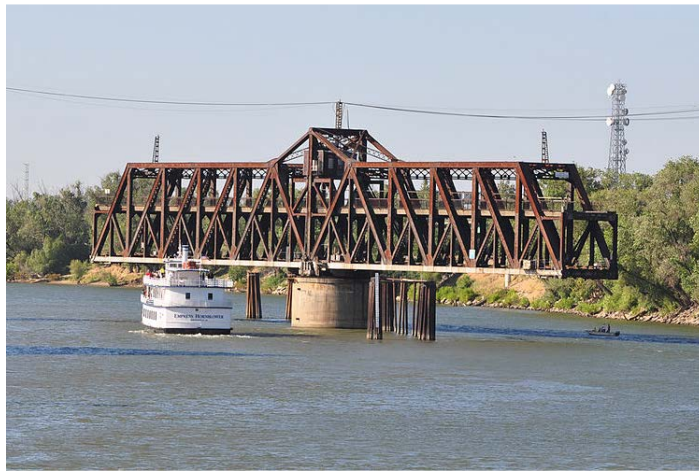
Figure 19 – I Street Bridge, Sacramento, CA
