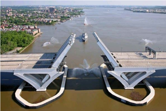
Figure 22 – Woodrow Wilson Bridge, Washington, D.C.
