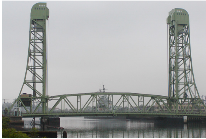
Figure 15 – Philadelphia Navy Yard Lift Bridge, Philadelphia, PA
