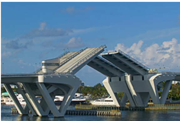
Figure 30 – 17th Street Causeway Bascule Bridge, Ft. Lauderdale, FL
