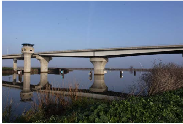
Figure 20 – Little Potato Slough Bridge, Terminous, CA
