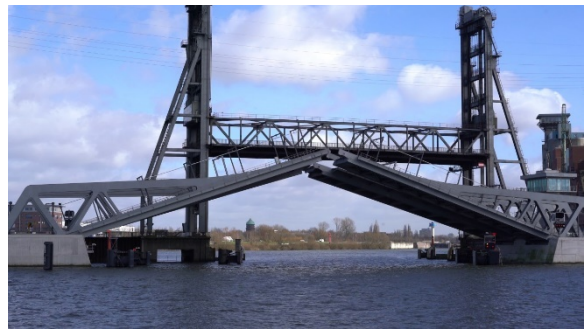
Figure 25 – Rethel Bascule Bridge, Hamburg, Germany (Front Bridge)
