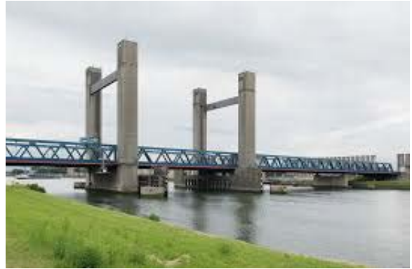
Figure 23 – Caland Bridge, Rotterdam, Netherlands
